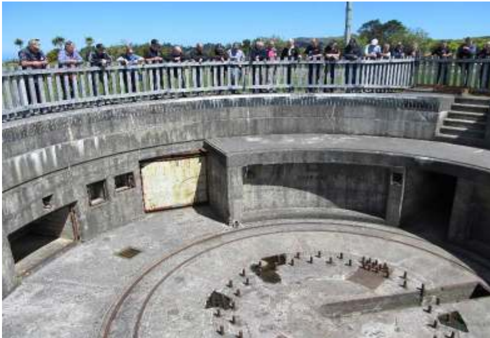
Looking down into where one of the guns was located
